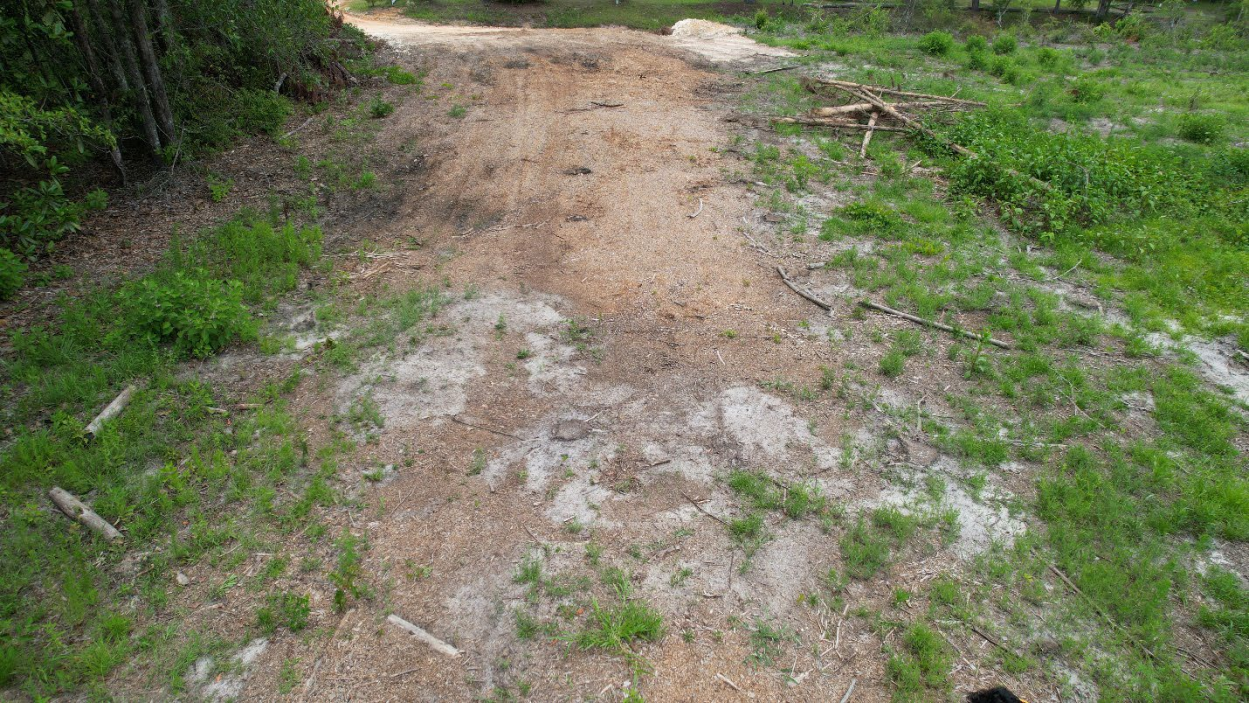
Image 8: Mulch application on forest roads to stabilize soil.
