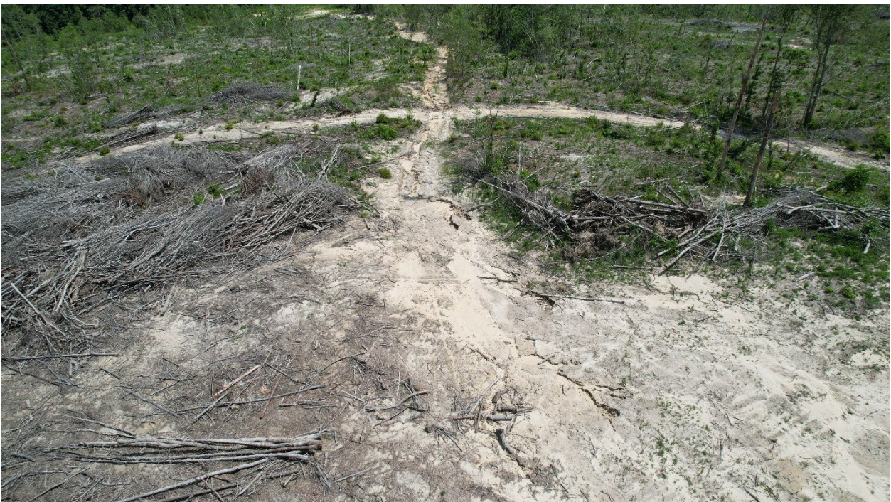
Image 2: Soil erosion on a forest road. Forestry BMPs were not followed in that no water diversion devices (waterbars and turnouts) were installed.
